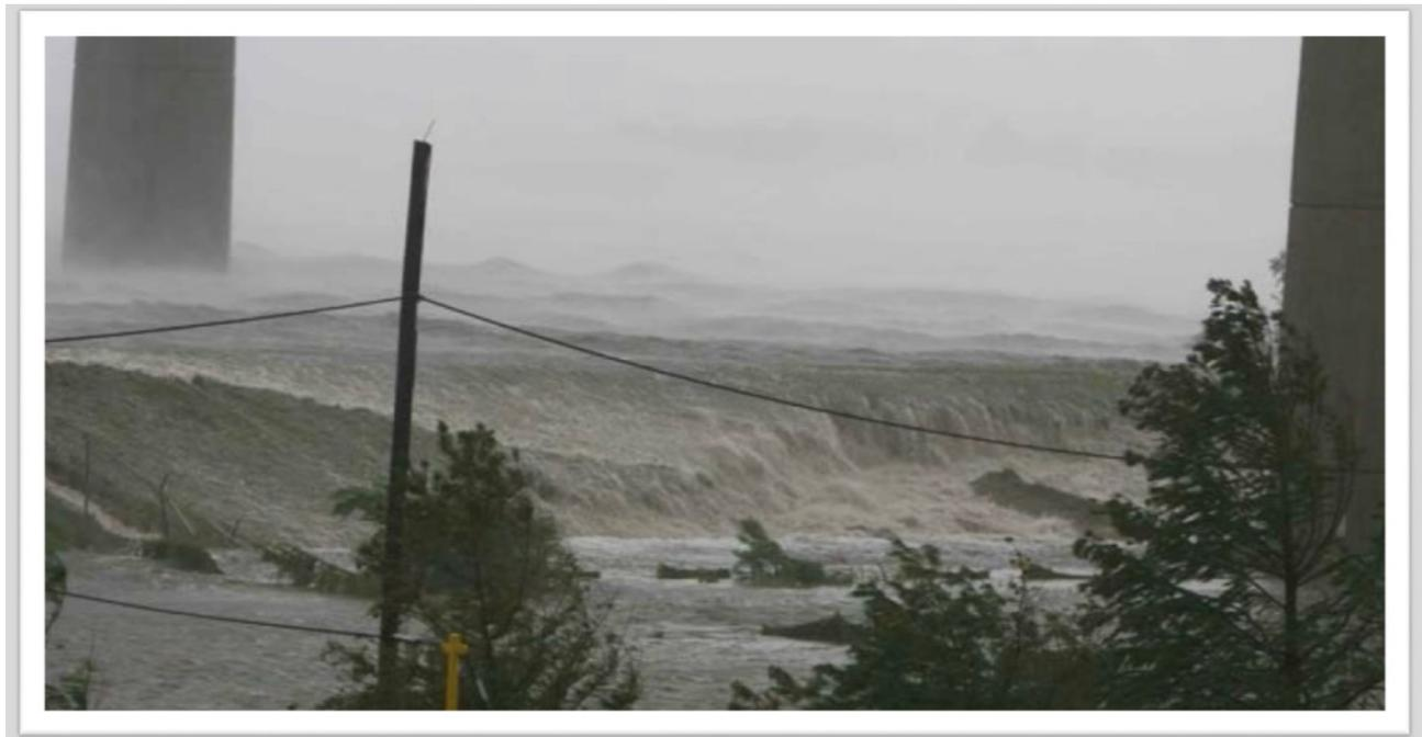
*Hurricane Katrina floodwater overtops a levee along the MRGO. Photo taken by an automatic camera installed at Entergy's Michoud power plant in New Orleans East.*
